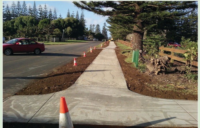
Airport to Burnt Pine footpath works
