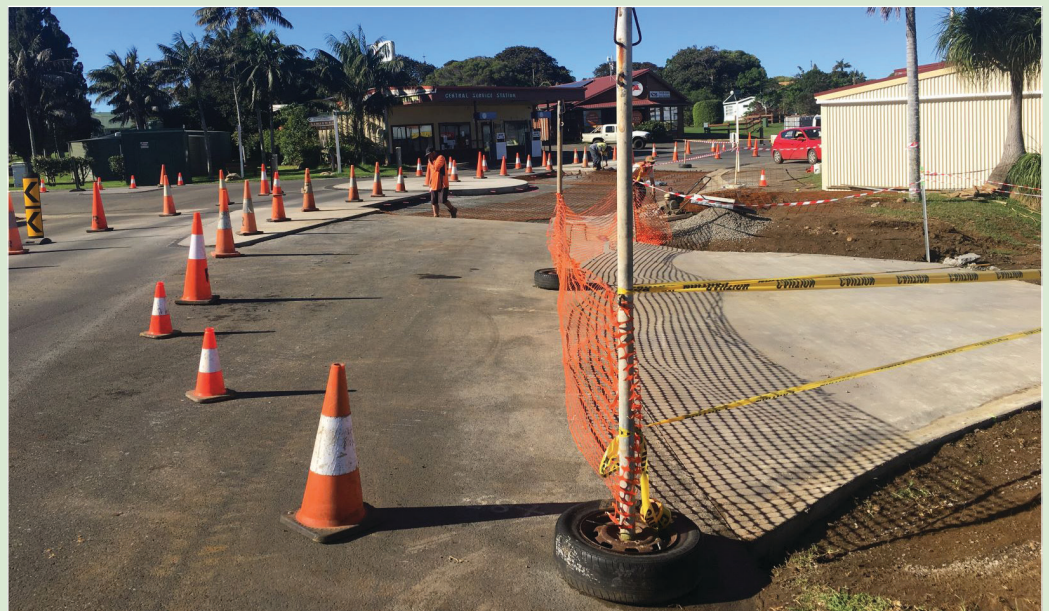
Roundabout works on the corner of Taylors Road and Grassy Road
