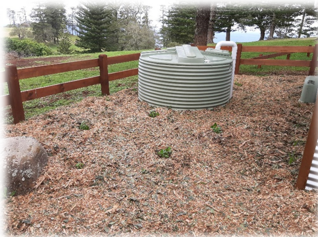
Before, during and after of the freshly planted toilet block at Puppies Point
