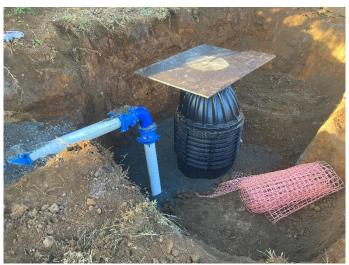
As a part of the footpath construction project from the airport to Burnt Pine, a manhole upgrade needed to be completed on Ferny Lane. The manhole was custom made with PE plastic. The plastic material is not affected by the gases of the sewage meaning that it will have an extremely long service life.
