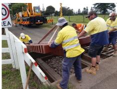
Each of the four town cattle grids are scheduled for replacement. As can be seen from the photos, each grid is constructed in two sections, at a cost of \$15,000 per section.
