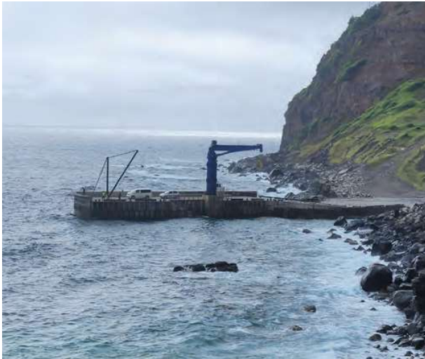
Kingston Jetty: NIRC made several steps to improve port and lighterage safety.
