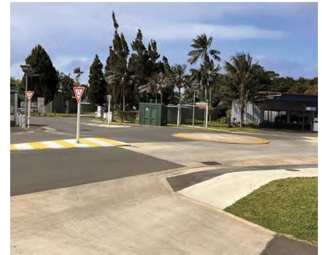
Footpath and roundabout improvements
