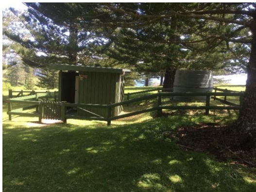
Figure 9. The Public Toilet at Puppys Point requires replacement
