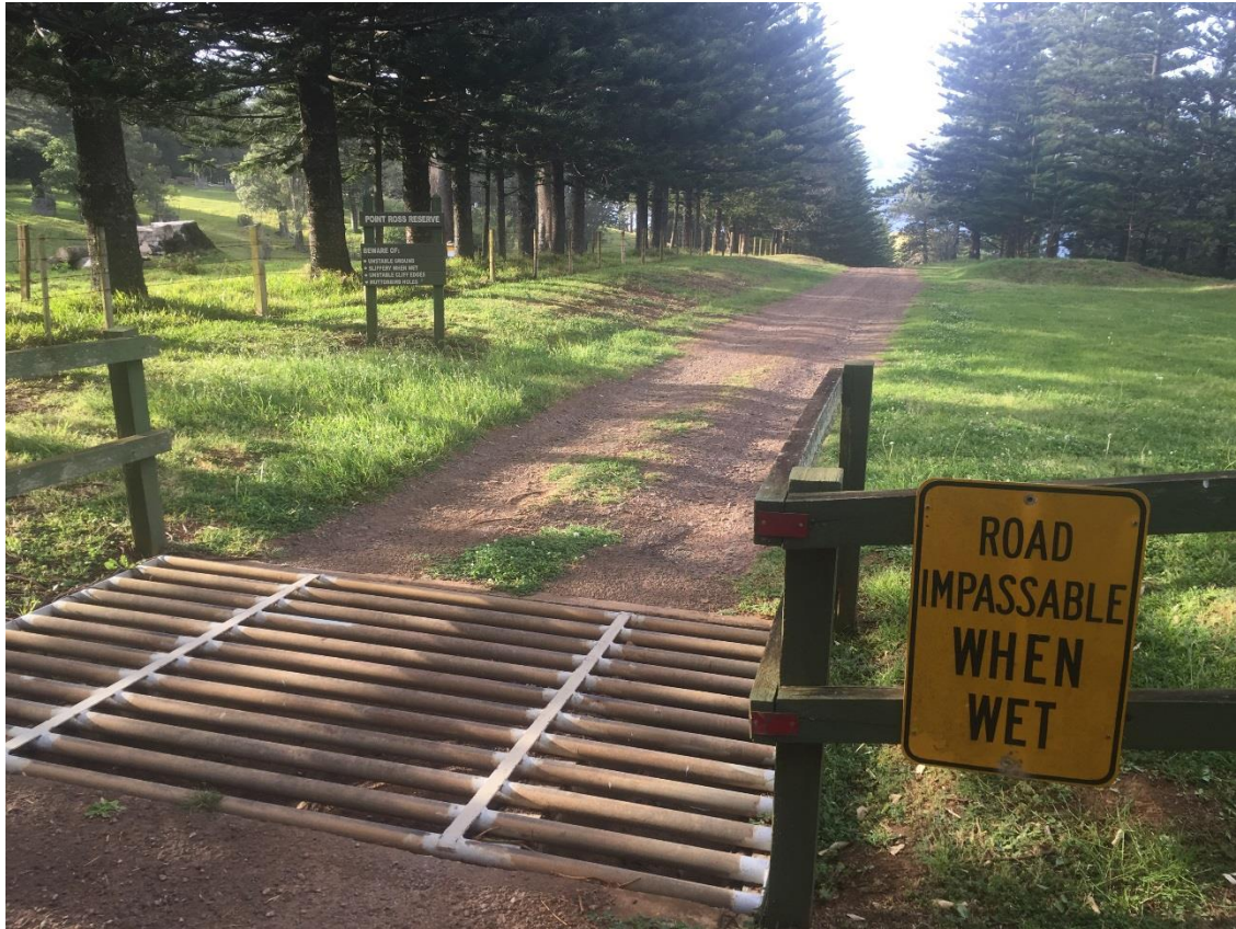
Figure 11. The dirt access road within the Reserve has been topped with gravel but is subject to potholing and gulying and can be impassable to two wheel drive cars in wet weather.
