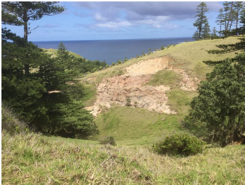
Figure 8. Looking East onto a westerly facing slope showing serious erosion and land slippage.
