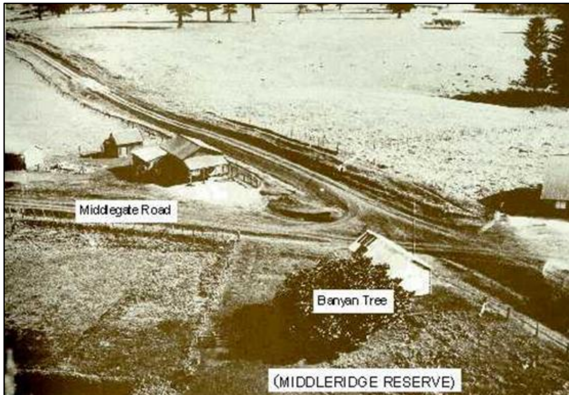
Figure 5: Early 20th Century View looking northwest over Barty Quintal's land at Middlegate
