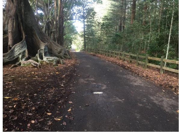
Figure 15: The timber post and rail boundary fence on new Farm Road.
