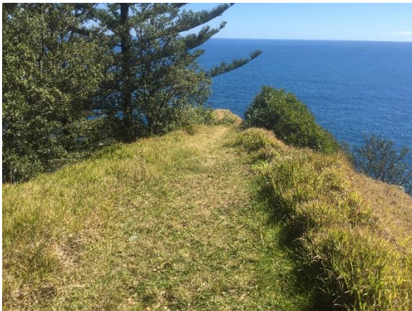
Figure 9. Public safety could be an issue in some areas, and barriers and signage should be installed to warn of the danger of steep cliffs in these areas.
