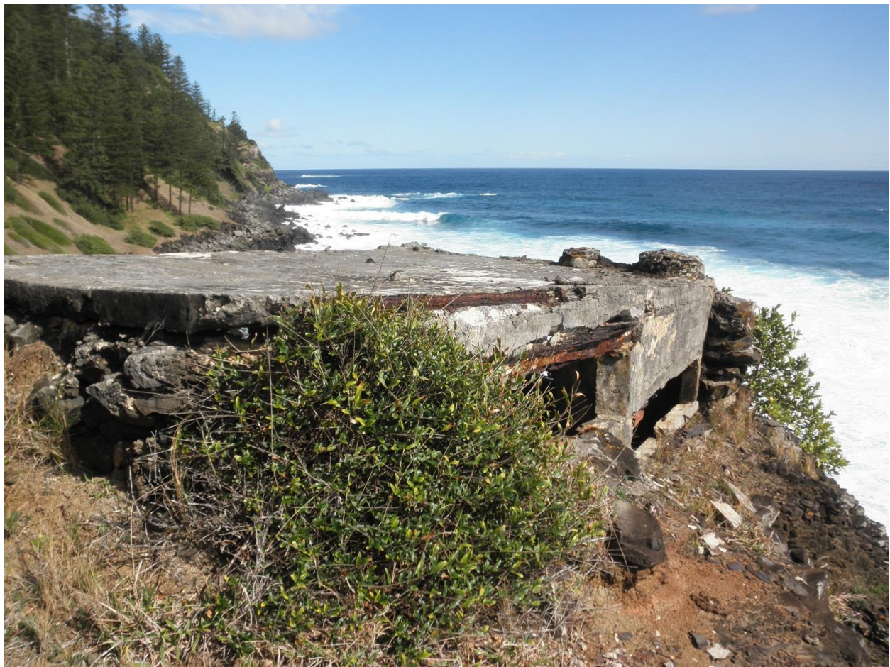
Figure 7: WWII Machine Gun Post, looking towards Selwyn Reserve.
