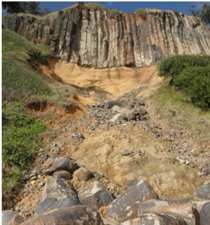
Figure 10: Rockfall from columnar basalt cliff above beach access track.
