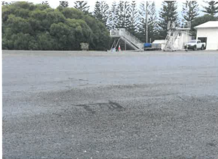
Figure 8 Photo example of depressions at Norfolk
