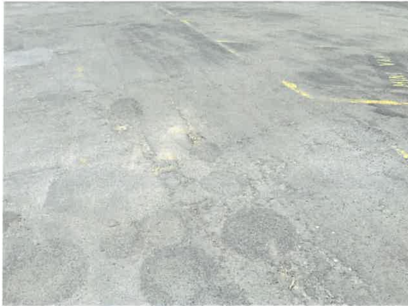
Figure 9 Photo example of landside car park surfacing quality
