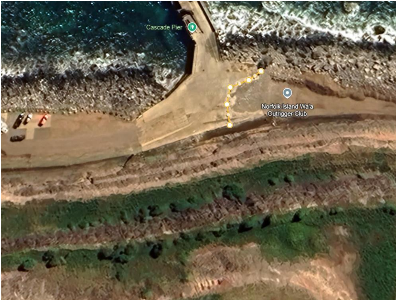
Figure 10 No public access past yellow mark line from the pier
