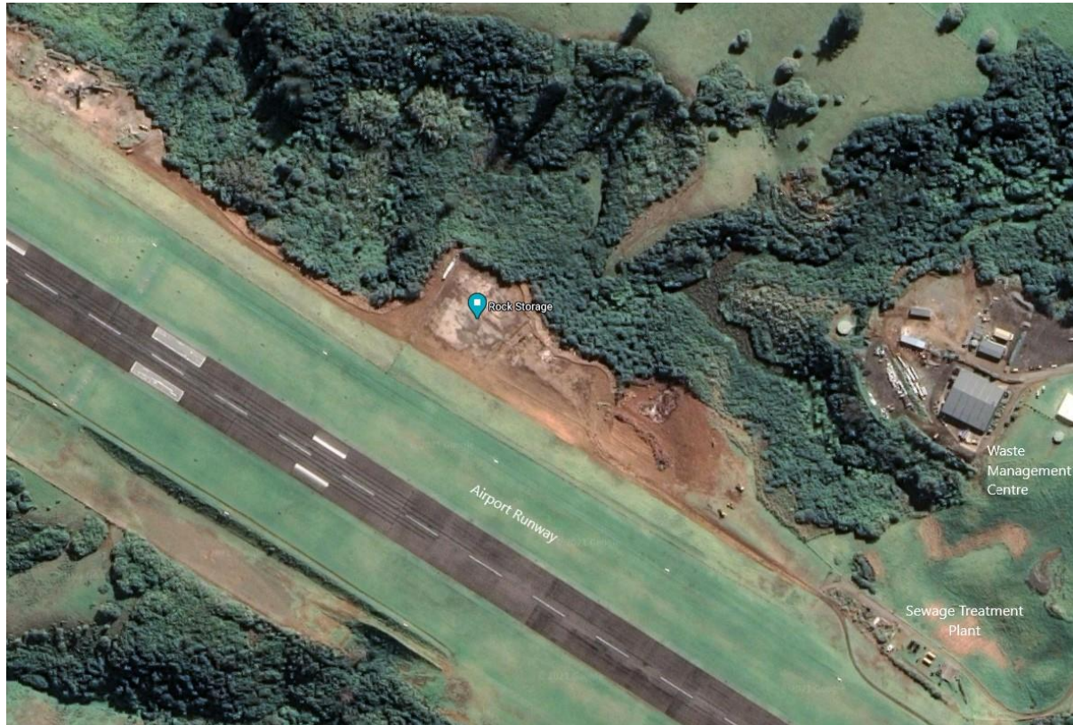
Figure 4 – Rock Storage location, Norfolk Island Airport Precinct
